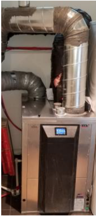
Conditioning Energy Recovery Ventilator (CERV) by Equinox uses a heat pump to recover heat while also providing supplementary heating, cooling and dehumidification. Earth tube up through slab to CERV
