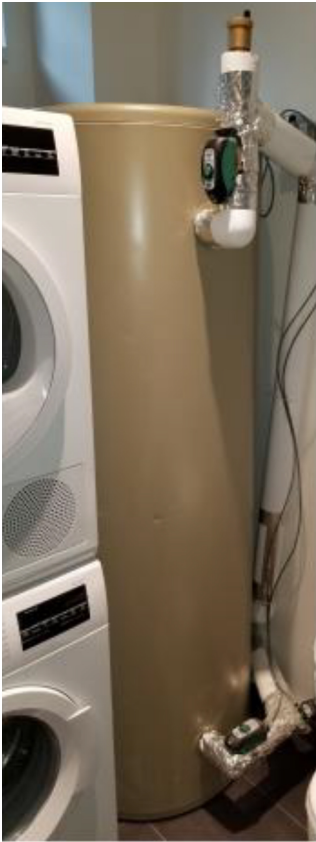
Sanden cold climate heat pump water heater uses CO2 as refrigerant to reduce greenhouse gases
