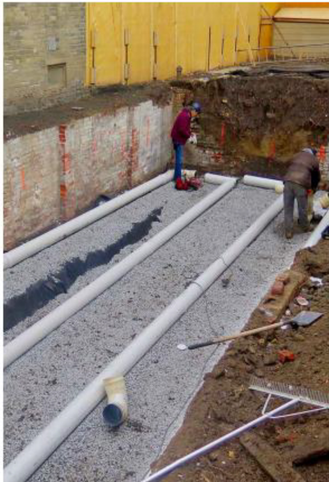
Earth tube underneath daycare play ground (right), preconditions fresh air into CERV ventilator
